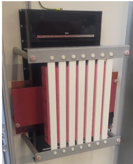
Figure 3.15 – HV Switch with DC storage frame.
