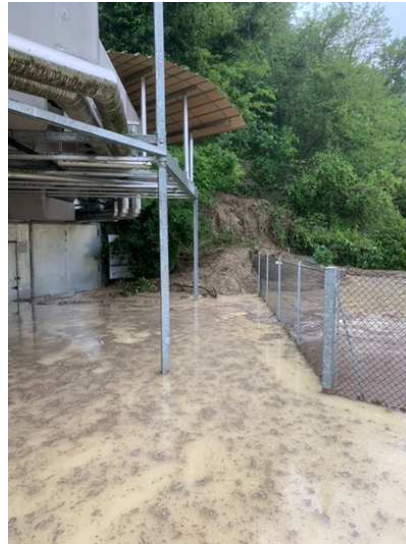
Fig. B.8 Flooding near the main entrance.
