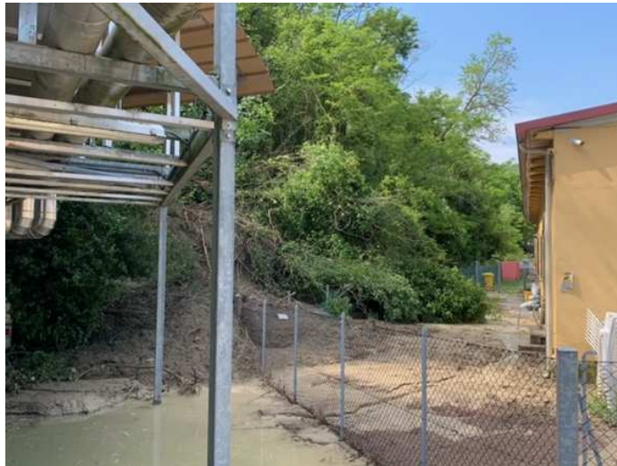
Fig. B.11 Obstruction of the corridor leading to the emergency exit.
