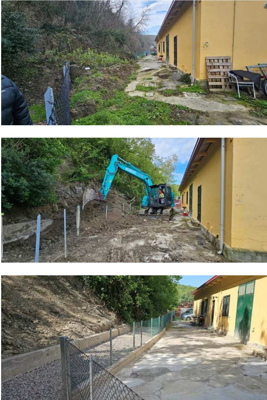
Fig. B.29 Removal of the landslide near the main entrance. Installation of drainage material and restoration of the fence.
