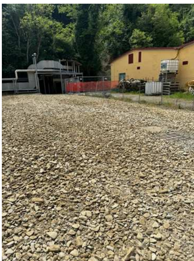
Fig. B.31 Removal of the landslide near the main entrance. Installation of drainage material and restoration of the fence.
