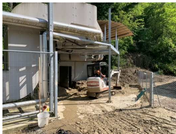
Fig. B.17 First clearance activities at the main entrance.
