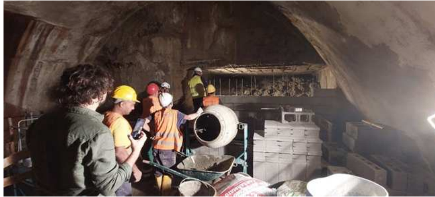
Fig. B.24 Restoration and closure of the landslide access in area 3.
