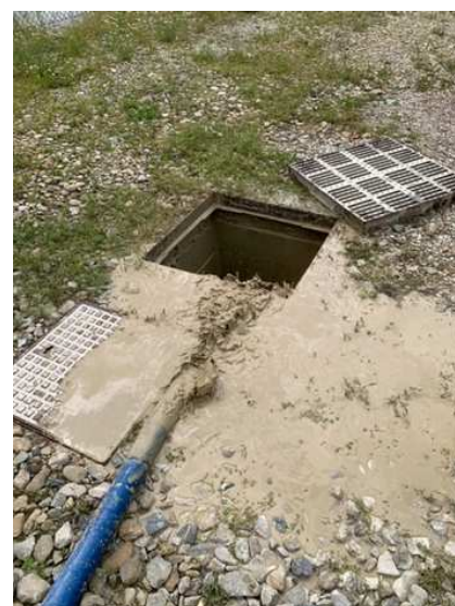
Fig. B.9 Mud removing operations using a water pump.
