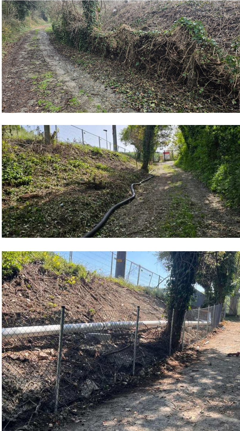
Fig. B.32 Repairing the drainage system
