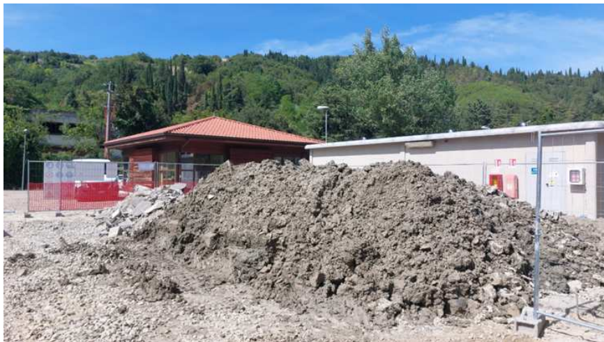
Fig. B.23 External deposit of mud and solid debris.
