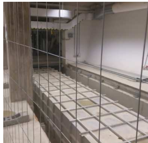
Fig. B.21 Recovery of return circuit placed in the cavity under the floor.
