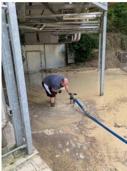
Fig. B.9 Mud removing operations using a water pump.
