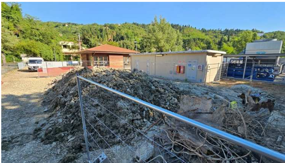
Fig. B.30 Removal of the landslide near the main entrance. Installation of drainage material and restoration of the fence.
