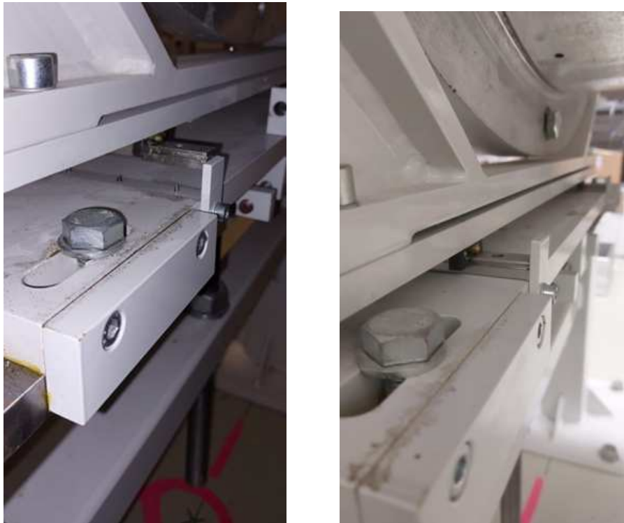
Fig. B.28 Repair of the pipe supports damaged by the lifting movement.
