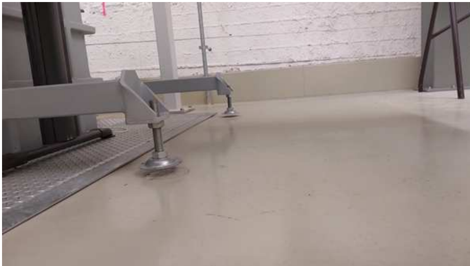
Fig. B.16 Lifting of the tunnel due to the floating of the wind tunnel.
