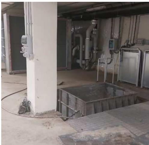
Fig. B.21 Recovery of return circuit placed in the cavity under the floor.
