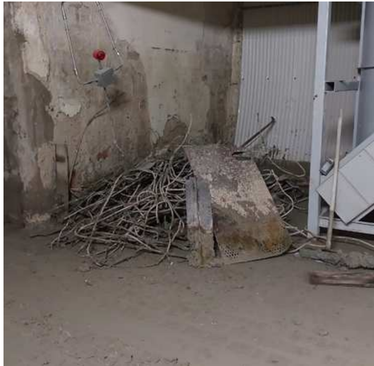
Fig. B.20 Removal of debris caused by the break-in of the separation wall.
