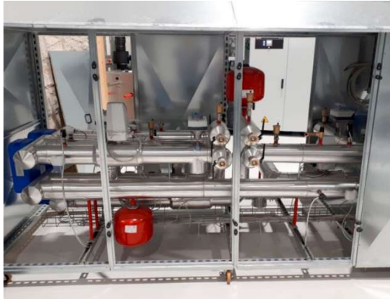
Figure 5. 7 Inside the substation and hydraulic connection to the Energy Exchange lab [152]
