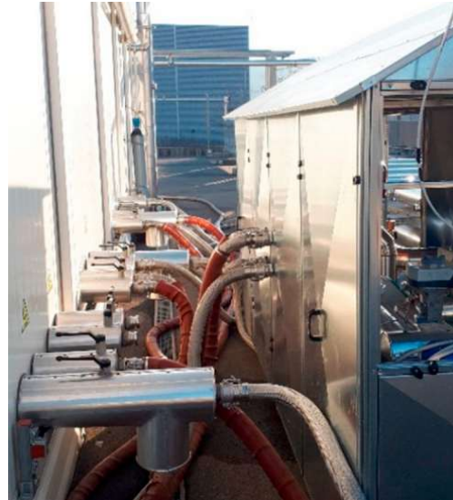
Figure 5. 7 Inside the substation and hydraulic connection to the Energy Exchange lab [152]
