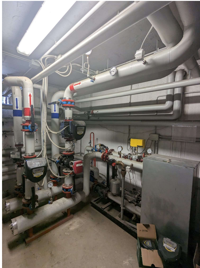
Figure B. 3 Focus on heat exchanger and the flow and return manifolds for RISC and DHW in the substation room
