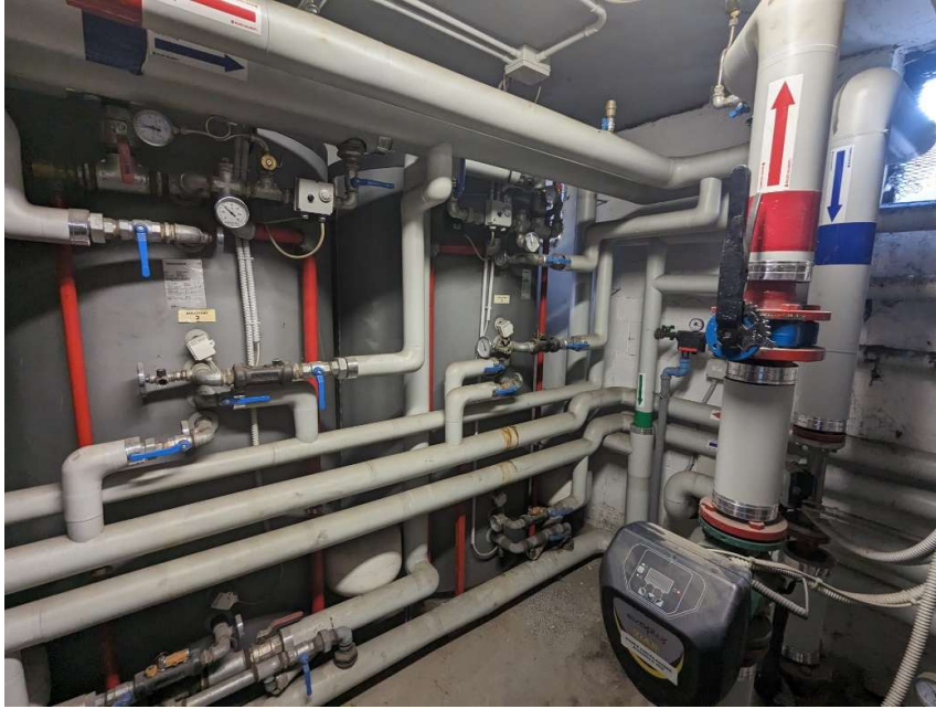
Figure B. 4 Focus on thermal storage system in the substation room
