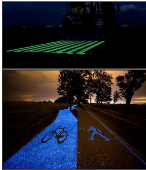
Figure 6-4: Strips with photo-luminescent paint
