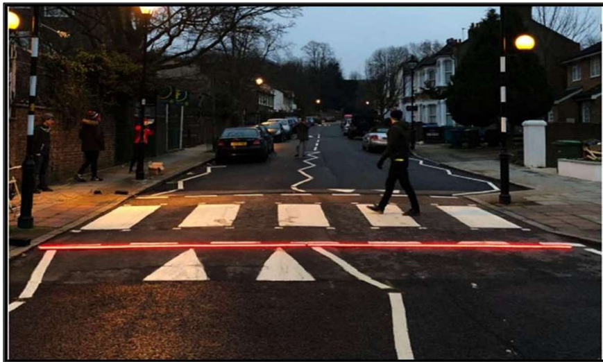
Figure 6-6: Crossing with line-of-sight system
