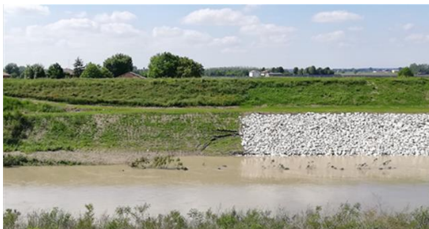
Figure 19 Deep-rooted plant planted on the Panaro river embankment close to Bomporto (Modena)
