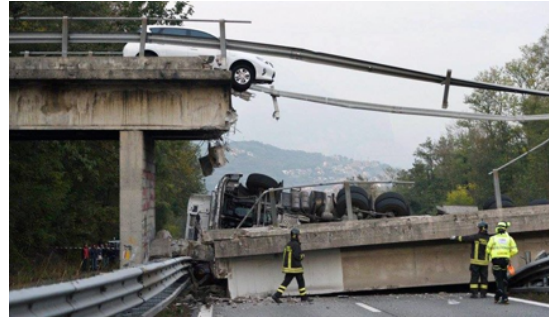
(b) Viaduct collapse in Lecco, Italy
