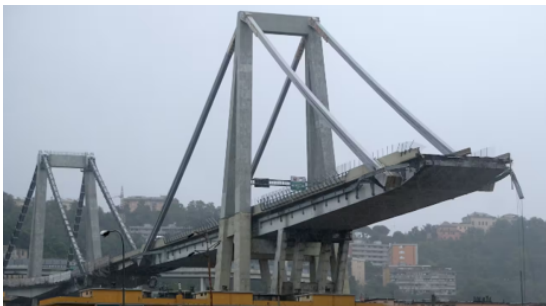
(a) Rest of the collapsed pier number 9
