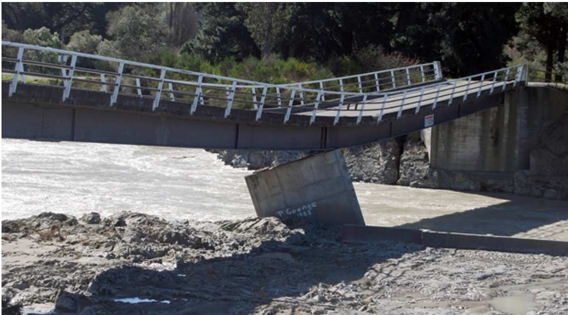
Figure 4.4: Example of a foundation vertical settlements
