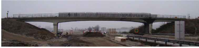
Figure 3.21: View of the S101 Bridge [218]
