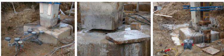
Figure 3.24: Photographic documentation of the pier settlement process [218]
