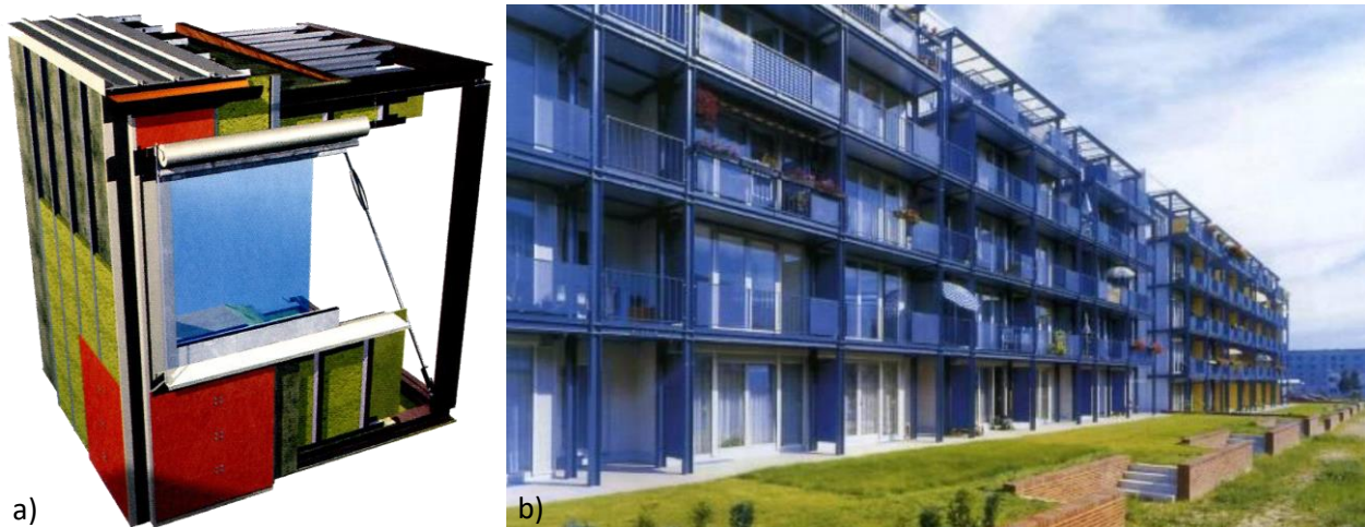
Figure 35 – a) Various possibilities on a single cell with the Structure/Cladding system; b) Retrofitting intervention of a Plattenbau in Leinefelde, Lessingstrasse (Germany), Stefan & Schnorr Architekten, 2000 – Source: [86]
