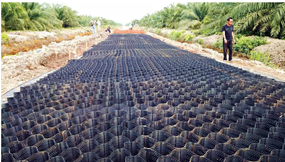
Figure 8 - Geocells used for fast access road building
