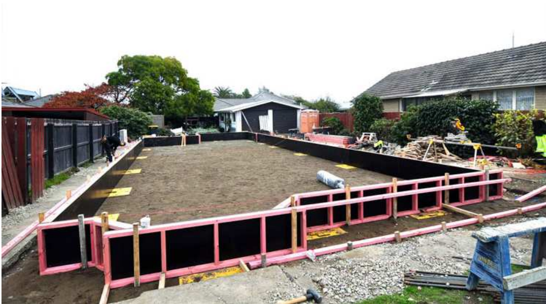
Figure 14 - Preparatory phase of the voided raft system: engineered base mat and jacking pads (courtesy of Cresco Engineering NZ)
