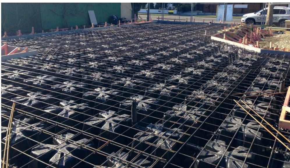
Figure 13 - Building phase of the voided raft system (courtesy of Cresco Engineering NZ)
