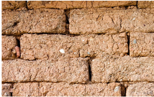
Figure 1.1: A combination of mud and papyrus dried into a construction brick in modern Egypt.
