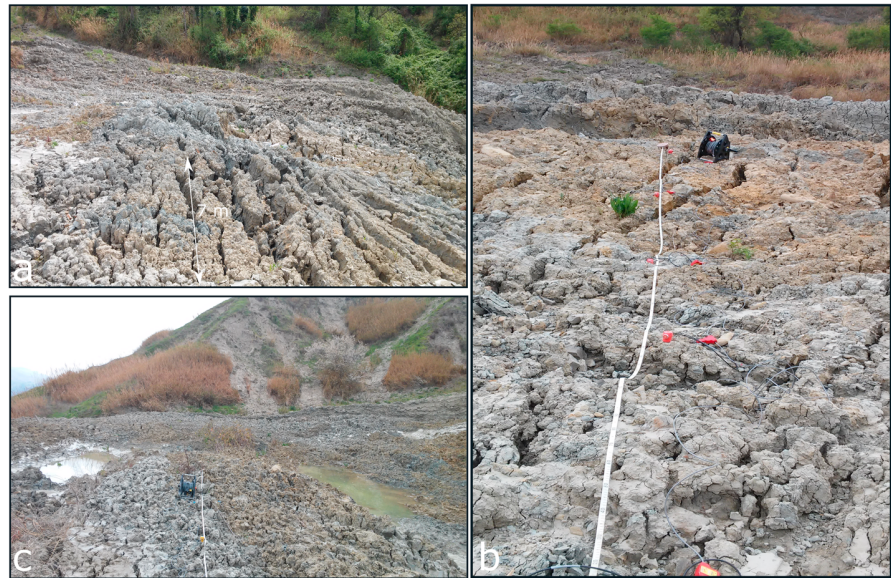
Figure 5. Photographs showing the difficult ground conditions encountered during periodic seismic surveys. (a, b) Cracks and open fractures characterize the landslide surface during the dry period; (c) water ponds and soft soil reduce the accessibility soon after a reactivation or an intense rainfall.
