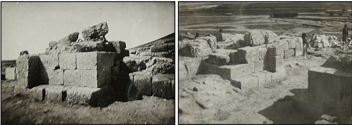
Figs. 2.58 - 2.59 - The western and the eastern towers of the Roman South Gate from northeast and from northwest, looking towards the outer city (CE Photo Album 2, Fol. 94, No. 920, Neg. 083695 and CE Photo Album 1, Fol. 256, No. 540, Neg. 033507).
