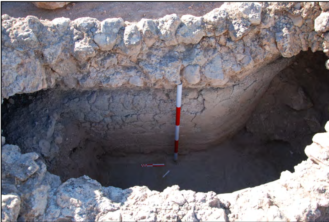
Fig. 2.122 - Detail of the Roman drain D.2600 in its western trait (D.2600c) where it was collapsed, with the inner plaster coating and calcium carbonate deposit. From southwest.
