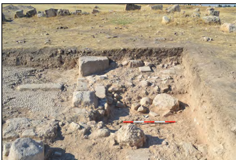
Fig. 2.109 - F.8904: collapse of the southern wall W.8903 inside the western room of the house. To the left is the wall W.8913. From north.
