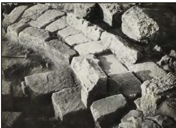
Fig. 2.62 - Roman gate: western wall of the eastern tower from north (CE Photo Album 1, Fol. 258, No. 543, Neg. 033510).
