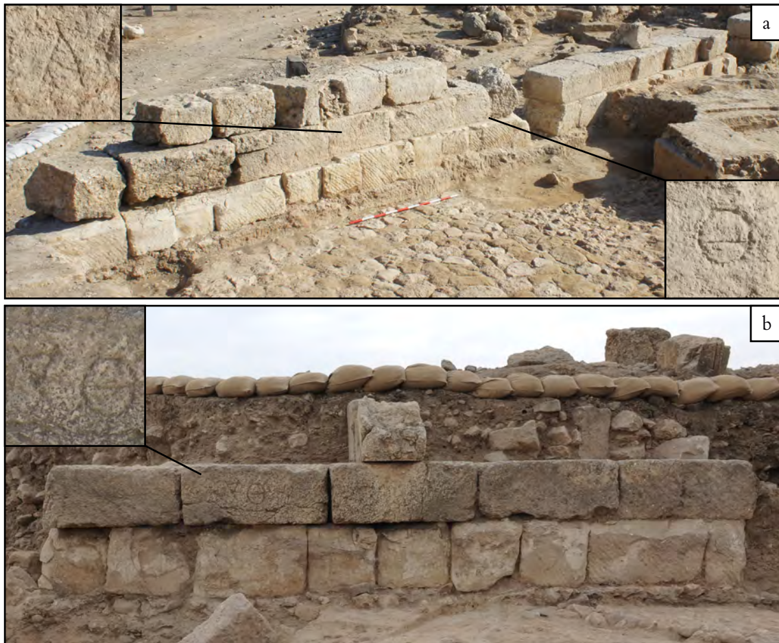
Fig. 2.39 a-b - Quarry marks engraved in the blocks of the foundation of W.2746. From south, in the westernmost portion and from north in the trait right east of it.
