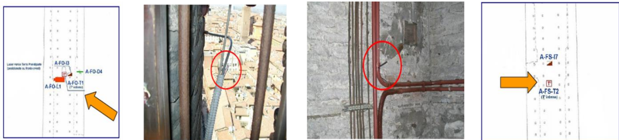
Figure 5-10: Thermometers installed on the Asinelli tower
