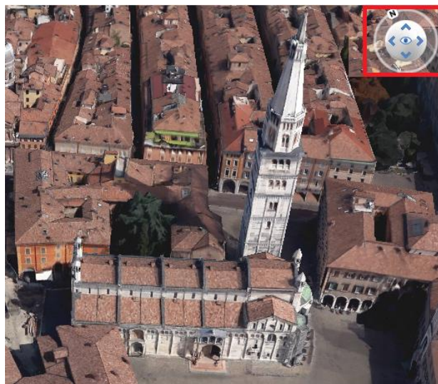
Figure 7-1: A three-dimensional (3D) view of the Modena Cathedral (Google Earth)
