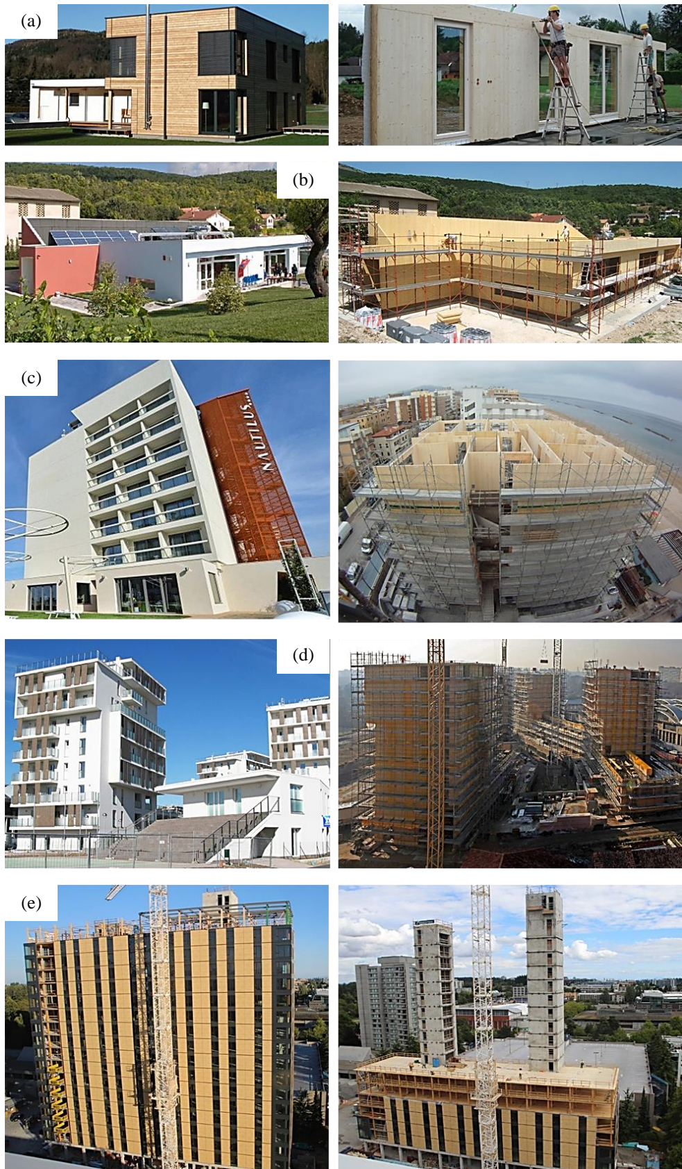
Fig. 2.17 Examples of CLT building: (a) Family house (Austria); (b) Kindergarten in Poggio Picenze (Aquila); (c) Hotel Nautilus, 7-storey (Pesaro); (d) Social housing-Via Cenni, 9-storey (Milano); (e) Student Residence Brock Commons, 18-storey (Vancouver)
