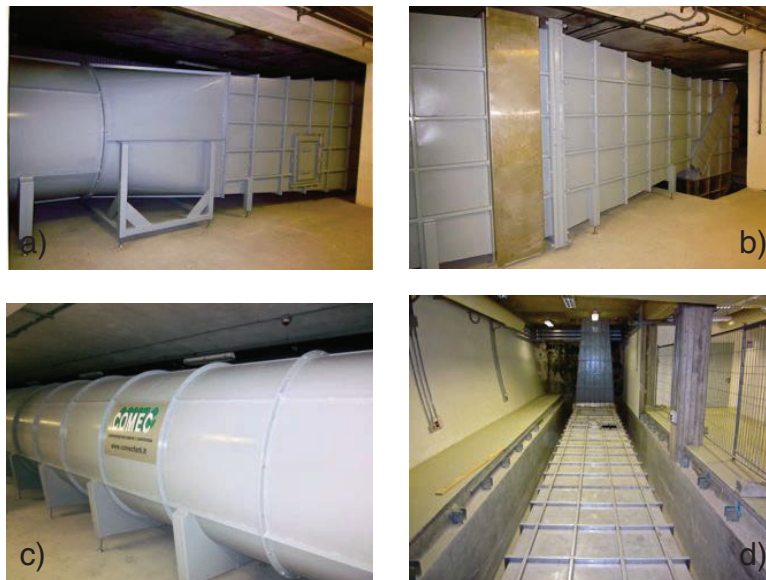
Figure 2.6: Elements of the return circuit. a) Rectangular to round shape converter after the heat-exchanger. b) Diverging section prior to the heat exchanger. c) Cylindrical elements of the return circuit. d) Section of the return circuit running under the floor prior to final assembly.
