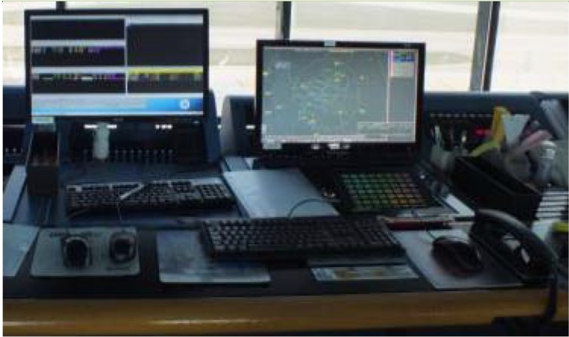
Figure 73. BOLOGNA AIRPORT CONTROL TOWER: COORDINATOR WORKING POSITION
