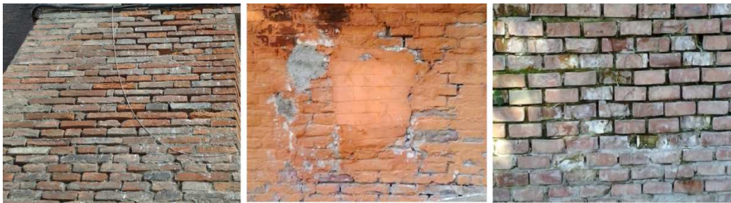
Fig.2. Examples of decayed masonries in need of repointing
