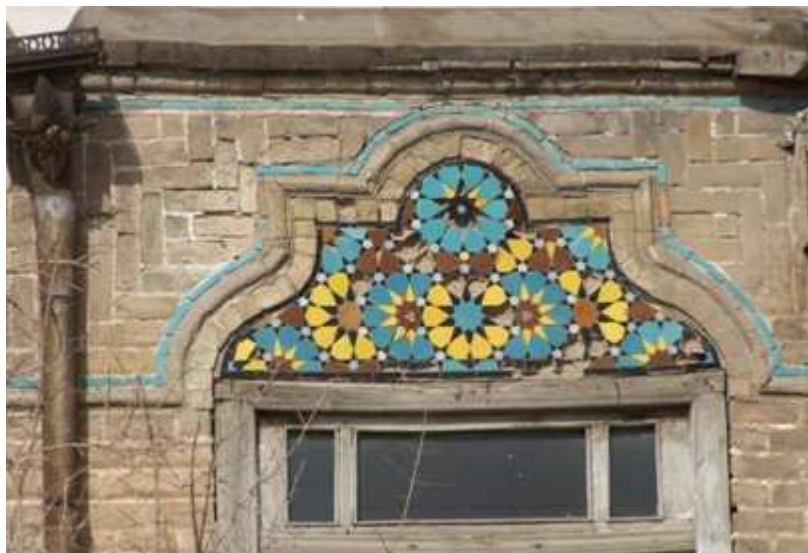
Fig. 50. A 20 th century house in Mashhad (north-eastern Iran) as an example of a national heritage element in need of repointing with sustainable binder
