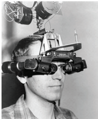
Figure 2.4: The “Sword of Damocles”, the first Head-Mounted Display by I. Sutherland and D.Sproull [Sutherland, 1968].
