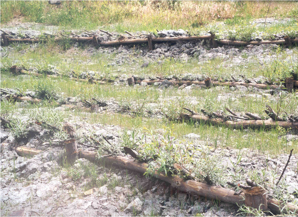
Figure 18. Soil bioengineering works at Vergato (courtesy of Cavazza)
