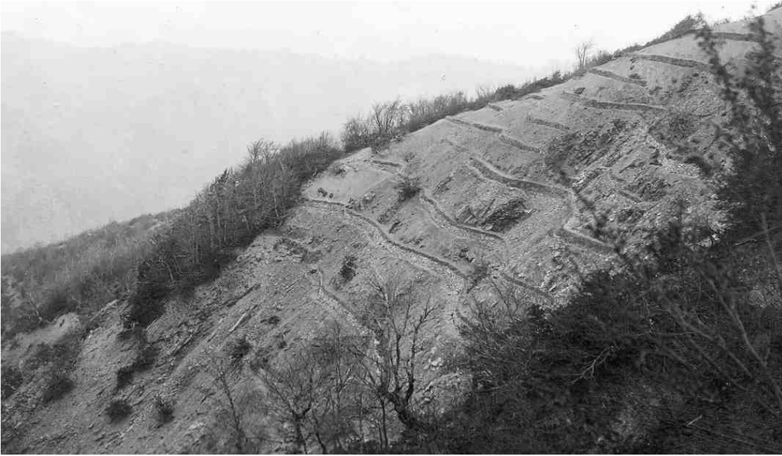
Figure 17. Terraces for reforestation, Porretta Terme, early '900s ( courtesy of Cavazza)
