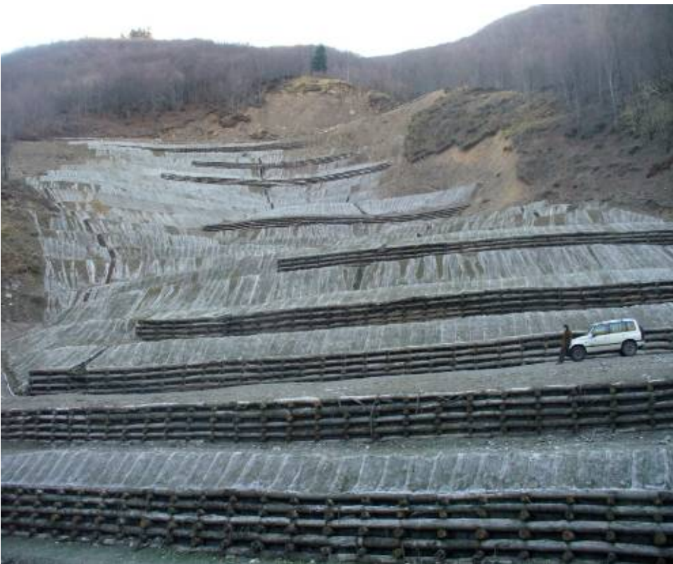
Figure 19. Log cribwall in Pracchia 2012 (Pistoia municipality intervention)
