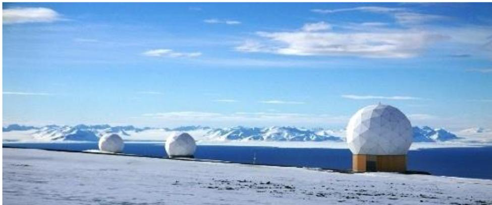
**Figure 45. The Metop satellites are operated via two CDAs collocated in Svalbard, Norway and linked to the operational ground segment in Darmstadt via fibre-optic and satellite communications links**
