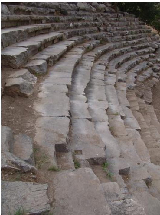
Cavity of awning (velarium) pole
