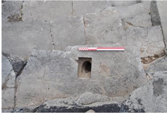
Cavity of awning (velarium) pole
