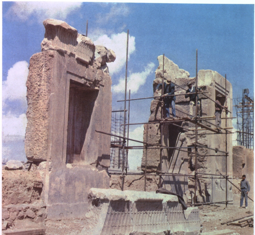
Figure 5.26. Persepolis: Consolidation of the stone parts in the Hall of a Hundred Columns in A. Tilia, Studies and Restorations at Persepolis and Other Sites of Fars , Roma, Istituto Italiano per il Medio ed Estremo Oriente, 1972.
