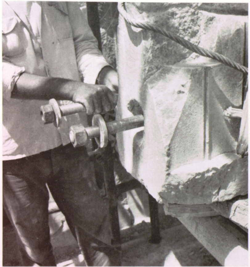
Figure 5.25. Persepolis: A cornice element in the Hundred Columns' Hall has been restored of many fragments, which have been attached with cement and held together by inserted steel bars, pulled from both ends by means of nuts turned on a spiral ridge, in A. Tilia, Studies and Restorations at Persepolis and Other Sites of Fars , Roma, Istituto Italiano per il Medio ed Estremo Oriente, 1972.
