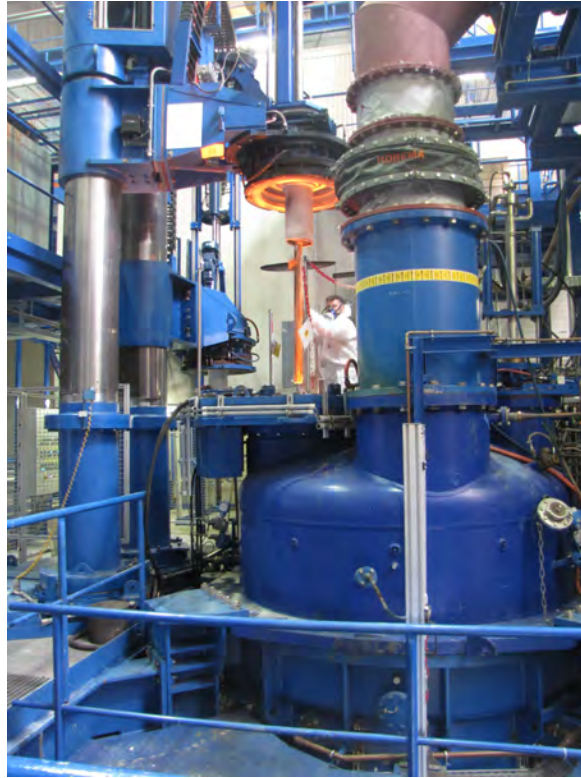
Figure 5.4: Maintenance work at the plasma torch at the GEKA Munster
