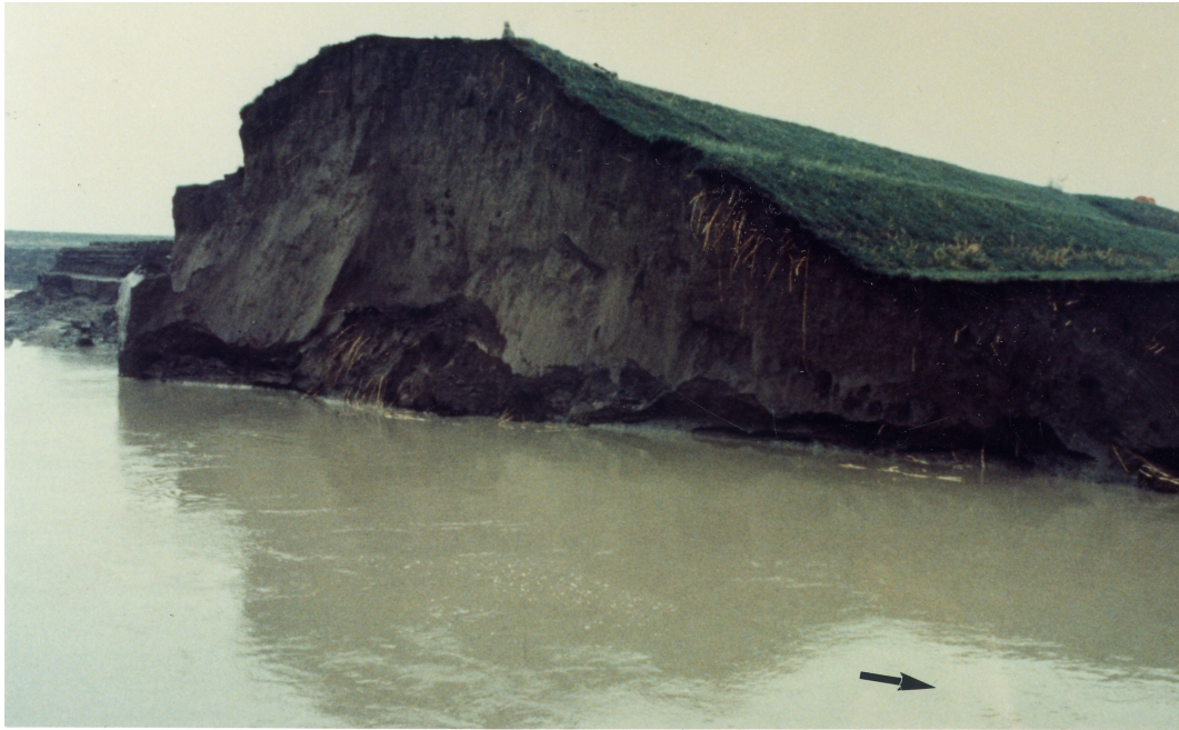
Figure 5.3: the breach before the beginning of repair works (27th of November). The overflowing water eroded the levee creating a 28m wide, 6m deep breach (Cremonini, 1994).
