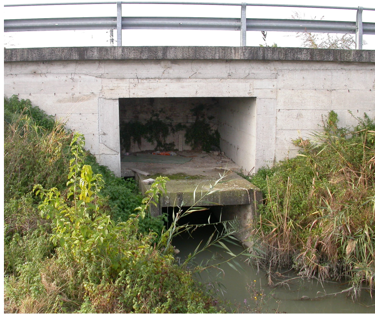
Figure 5.5: box culvert connecting San Prospero drain and Riolo drainage channel; the culvert passes under the levee of the latter.
