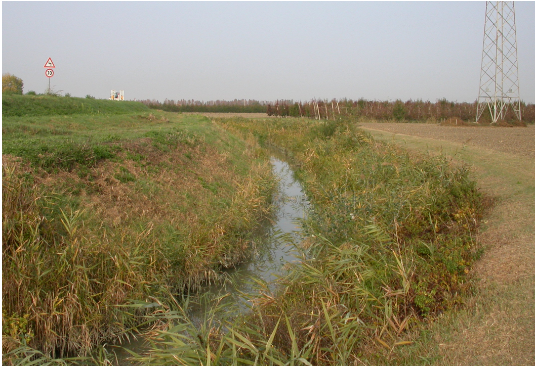
Figure 5.2: the San Prospero drain near Malabergo; the roughly triangular cross section is 10m wide and 3.3m deep; on the left side the levee of the Riolo drainage channel is visible.
