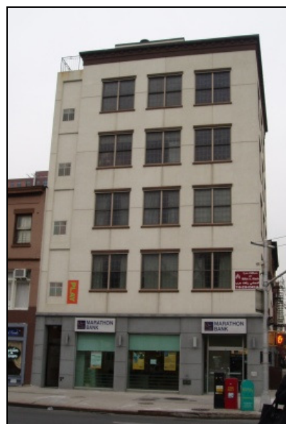
Figure 10.35. – The building today Source: photographed by the author
