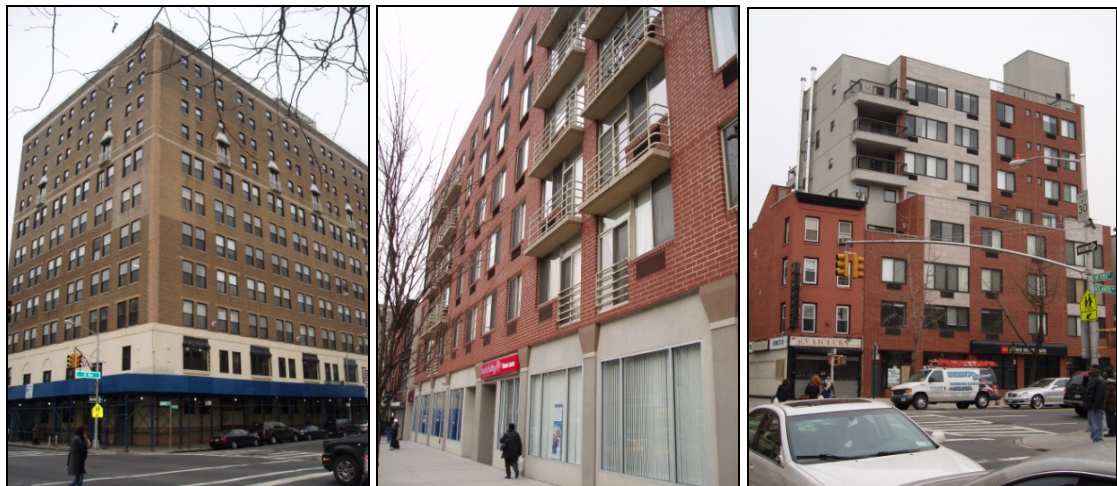
Figure 10.23. – Twentieth and twenty-first century commercial residential building type Source: photographs of the author
