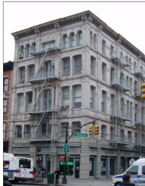
Figure 10.33. – The building today Source: photographed by the author, 2010
