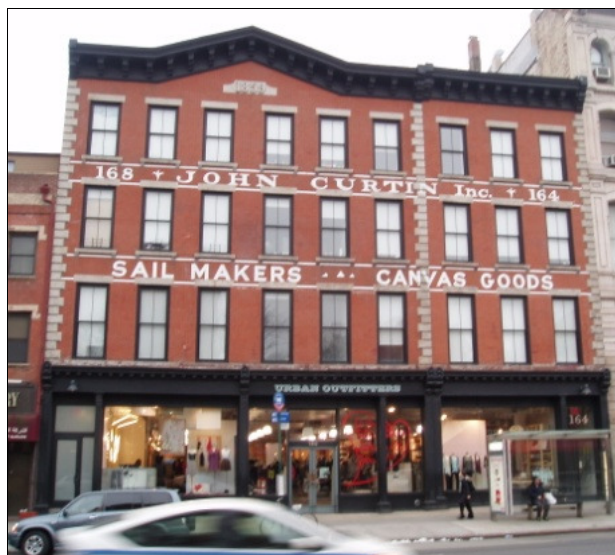
Figure 10.27. – Sail Makers mix commercial residential building Source: picture of the author, 2010
