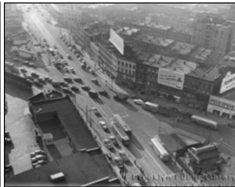
Figure 10.11. – ATURA site in 1960s Source: Brooklyn Public Library
