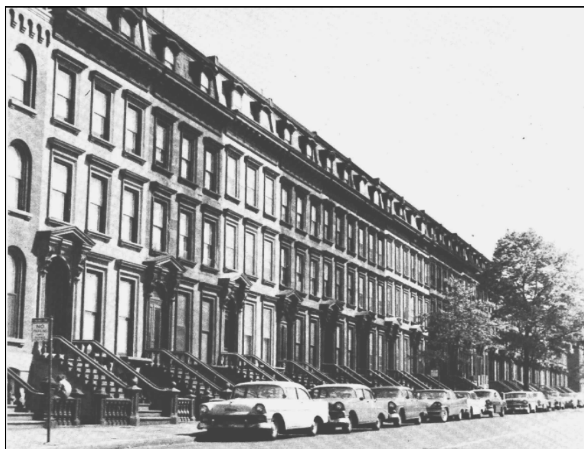
Figure 9.16. - Brownstones built in the 1890s as one family residence and converted into multi-family buildings for the poor Source: Reynolds, 1893
