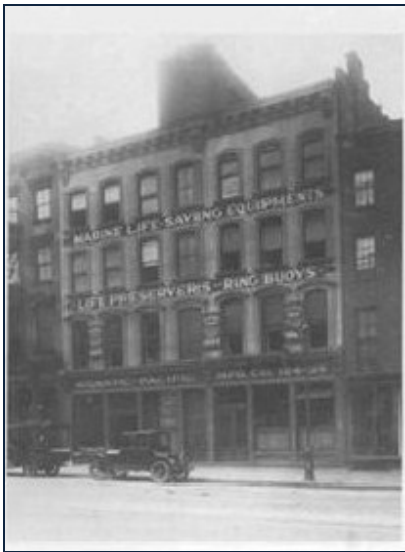
Figure 10.24. – Atlantic Pacific Building Source: Brooklyn Public Library, 1950s
