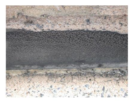
Figure 3.4. Centennial Hall, black thick crust in area protected from rain run-off.
