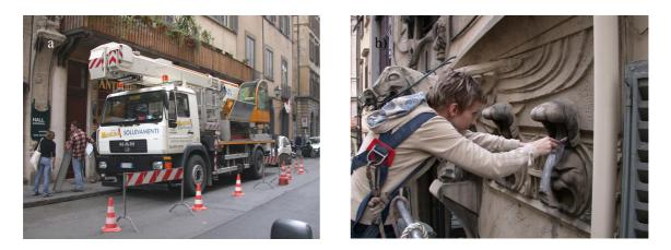
Figure 3.9. Sampling: (a) platform lift, (b) collection of the black crust from area protected from rain ran-off.
