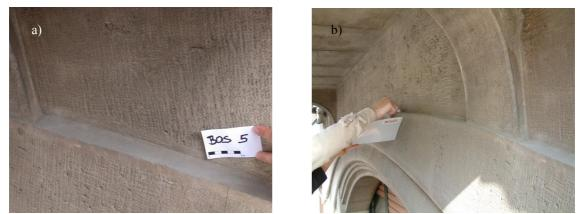
Figure 3.11. Casa Galleria Vichi. Sampling point, (a) and (b) incoherent grey deposit, easily collected by brush
