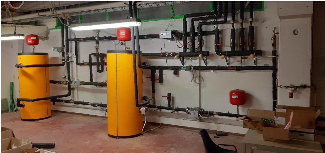
Figure 2.18 – View of the test ring inside the laboratory.
