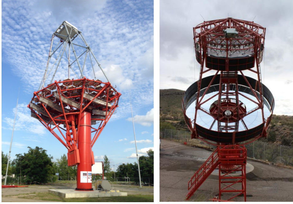
Figure 1.7: The MST design explores two different concepts. On the one hand, inspired by HESS and VERITAS current observatories, a 12 meters diameter modified Davis-Cotton (DC-MST) optical layout and a PMT camera. On the other, a novel 10 meters diameter Schwarzschild-Couder (SC-MST) optics incorporating a novel Silicon Photo-Multiplier (SiPM) camera. Credits to [Bar20].
