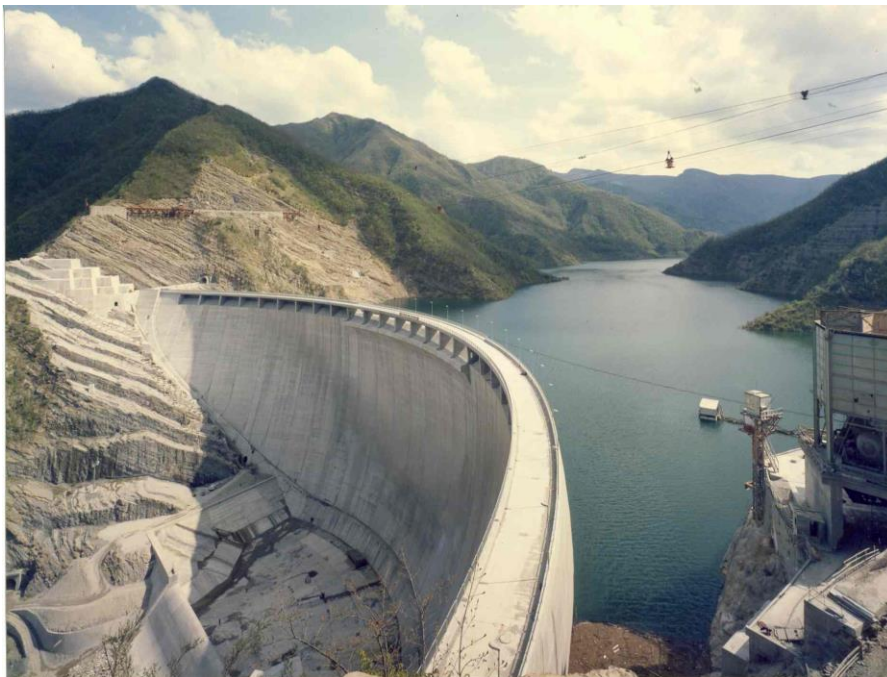
Figure 1.2. View of Ridracoli Dam in 1982, at the end of construction works (courtesy of Romagna Acque – Società delle Fonti S.p.A.)
