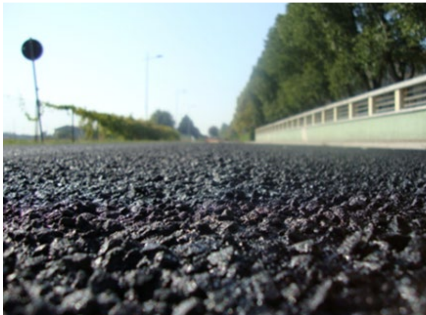
Figure 12. Cold laid acoustic microsurfacing in an Italian experimental site [73].
