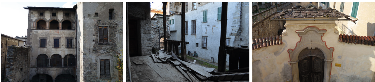
Figs. 56-58. Chiuro. Some of the topics investigated: porticoed courtyard of Palazzo Besta de' Gatti; wooden loggia; stone portal
